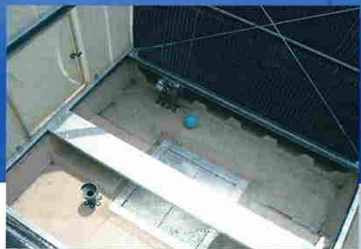
Lower water basin
